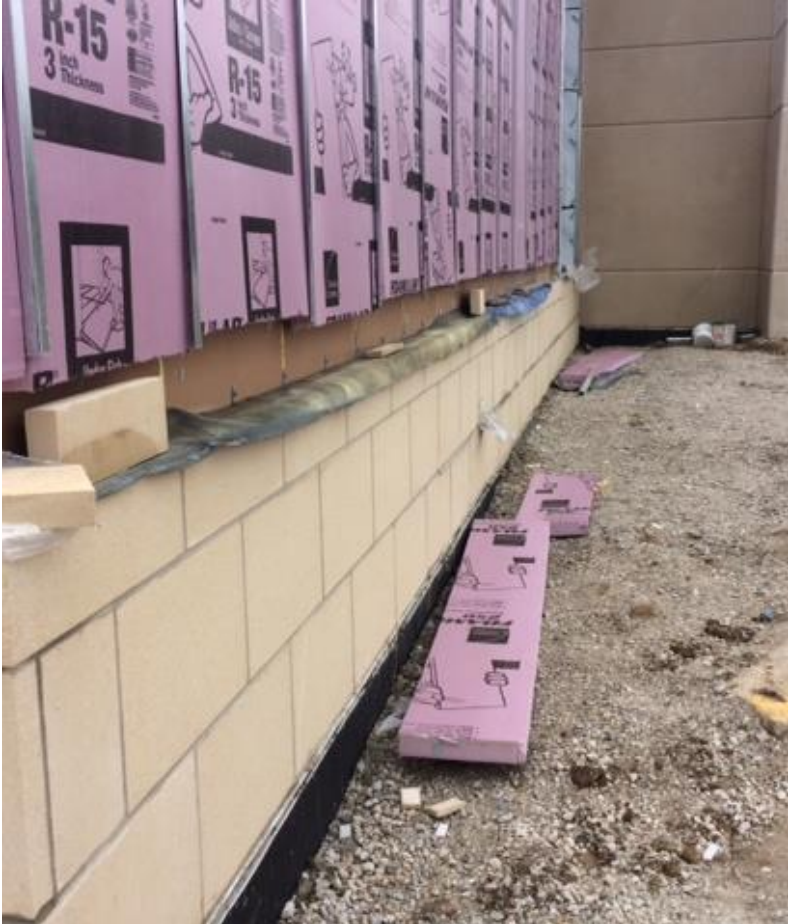
Exterior finish work underway on west side of new addition along State St. This is the stone veneer "skirt" which will run the length of the precast walls which aren't finished and along some areas of the existing school.
